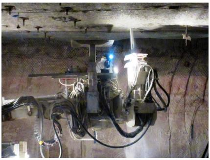
An Underground Operations employee, wearing anti-contamination clothing and a respirator, installs bolts in Panel 7 of the WIPP underground.
